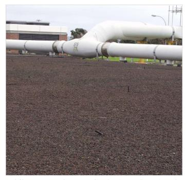
Earth filter No. 5 treats odorous gases from the primary sedimentation tanks. The fibreglass ducting extracts foul air from the primary tanks and passes it to the filter bed.
