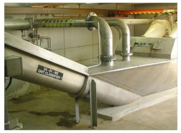
Incoming screened sewage is sent to one of 12 grit removal tanks which are at the head of each primary sedimentation tank.
